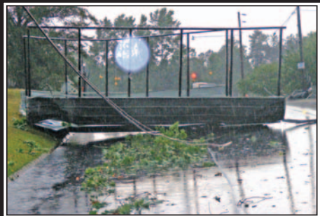
Pardon me, have you seen my carport? This carport ended up laying upside down on the road in Lilesville.
